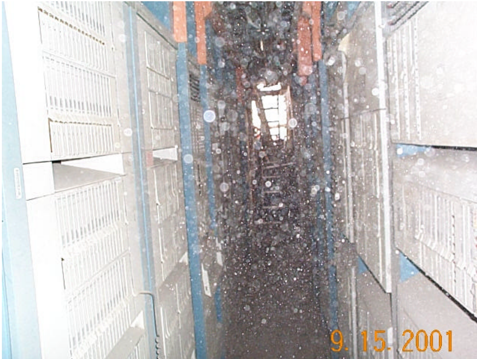
DACS III & IV Spots on the lens are from dripping water from above. Note hole in wall At the end of the isle.
