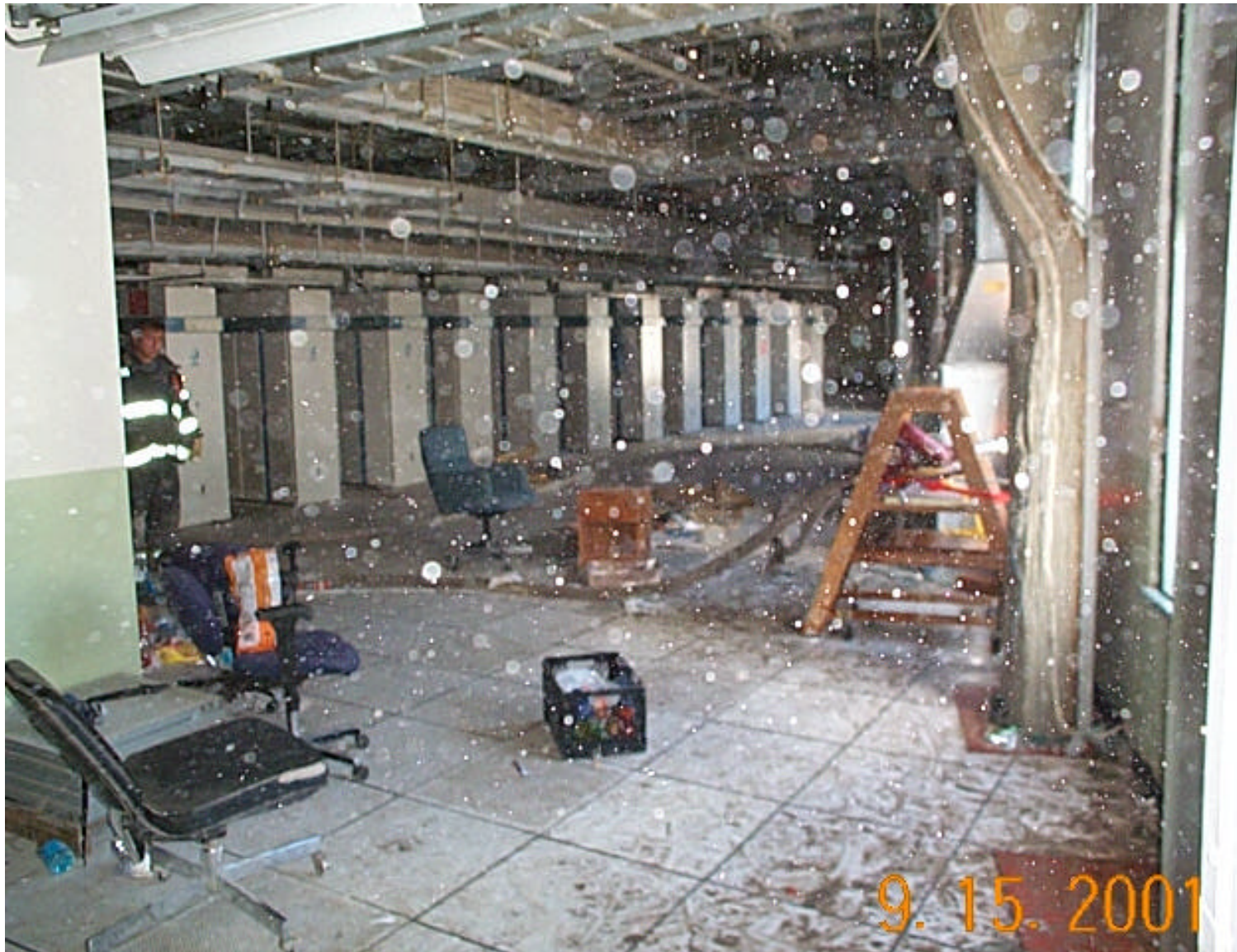
5ESS on 7 th flr. Note fire hose in ladder at window. Spots caused by water spraying around.
