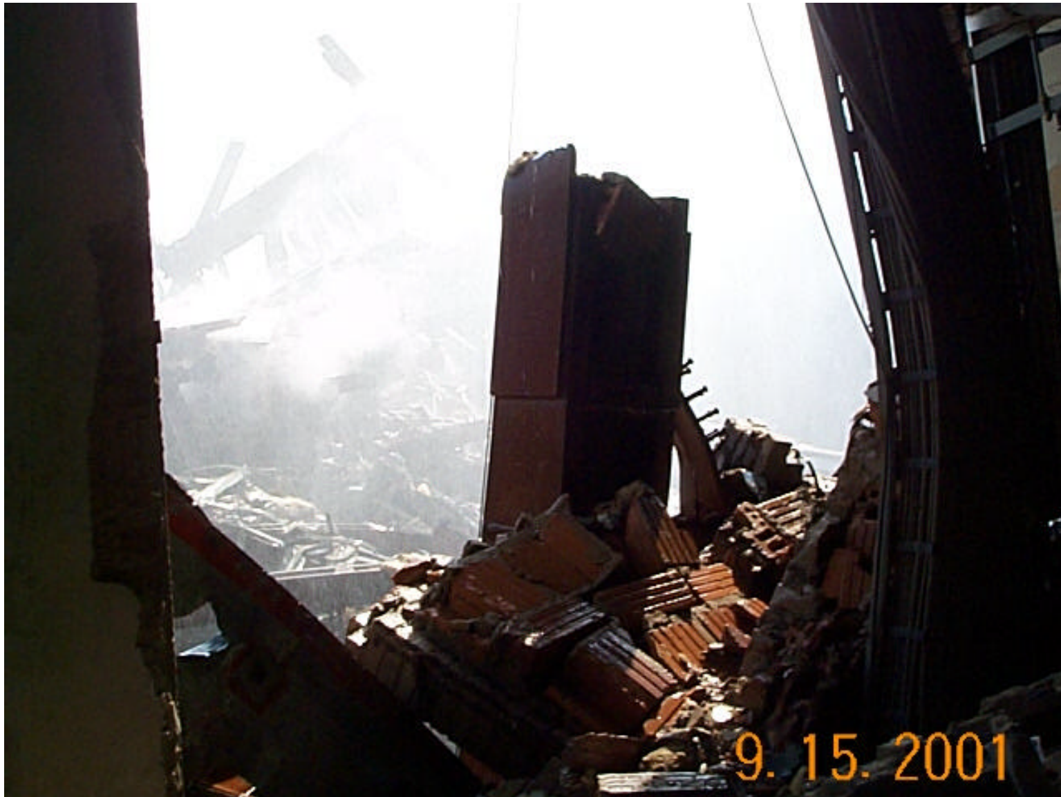
Looking out the southeast corner of 140 West Street. DACS and Access equipment on the right.
