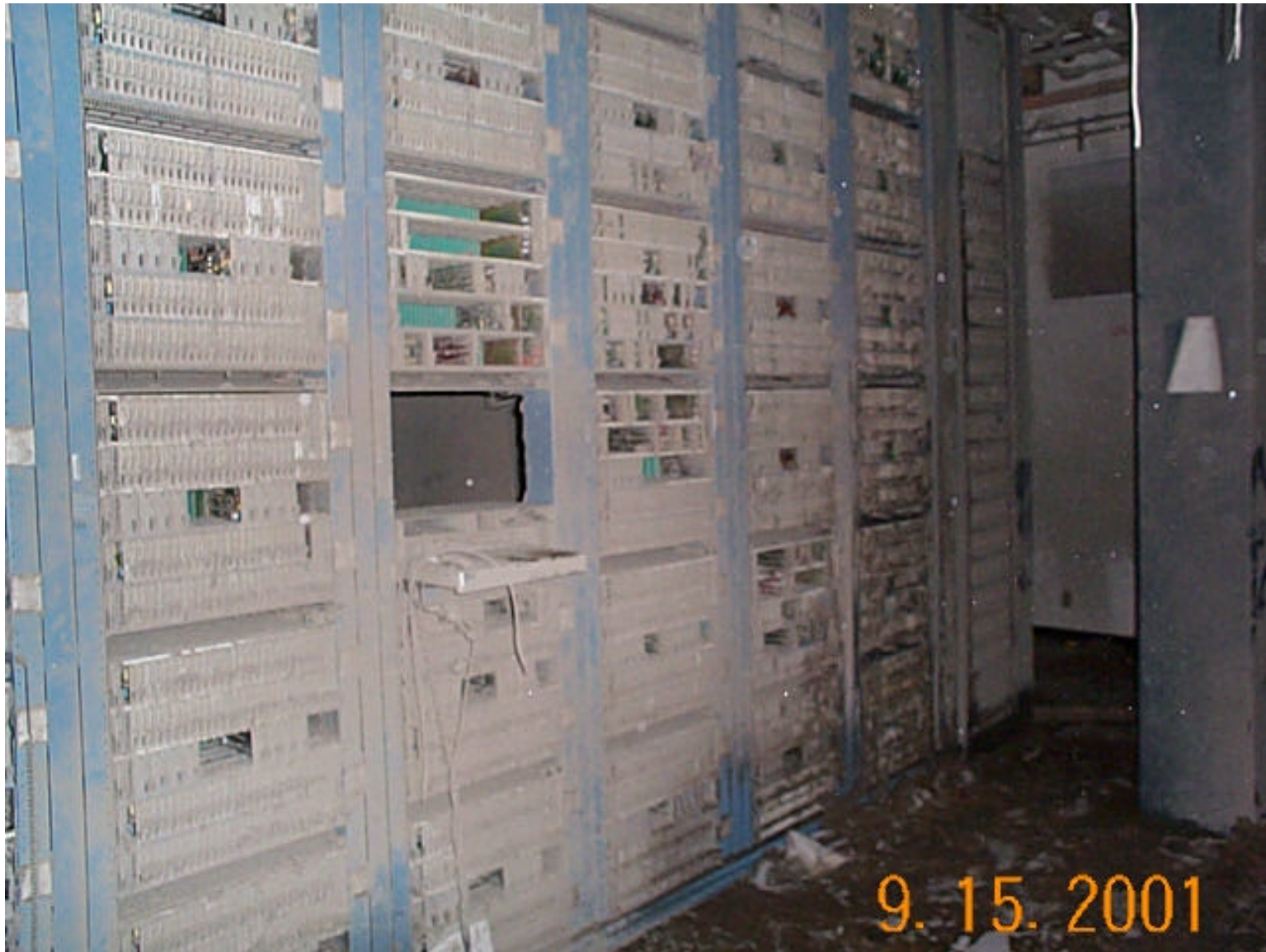
Access equipment 4 th flr.
