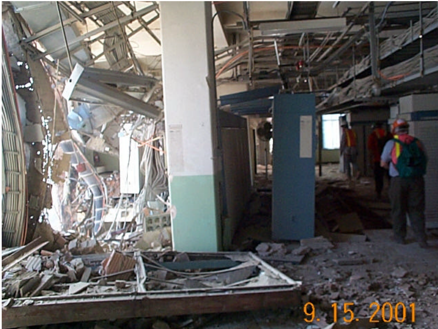
5ESS on the 7 th floor in the southeast corner.
